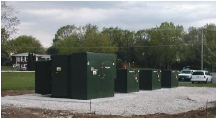
Utility substation placed in the middle of a suburb without the need for fencing and overhead lines
