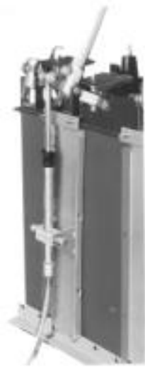
Remote cable operator connection to switch tank and operating handle.
