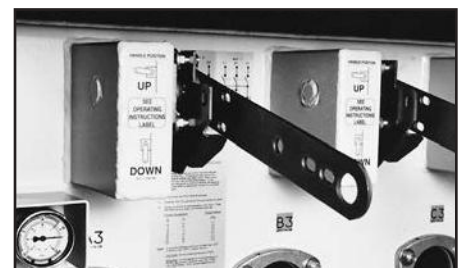
▲ Single phase interrupter operating handles.
