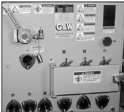
▲ Switch with front mounted fusing.
