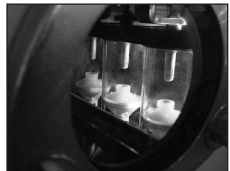
▲ Load break switch visible break
