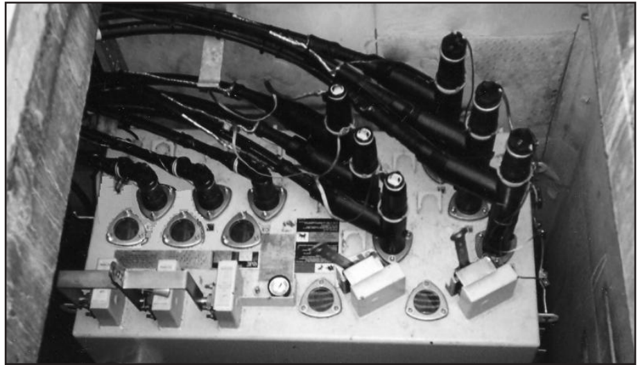
▲ Model VPVI with three phase interrupter operating handle.
