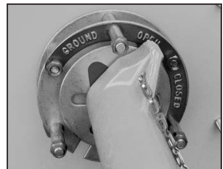
▲ Load break multi-position switch operator.
