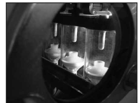
▲ Load break switch visible break.
