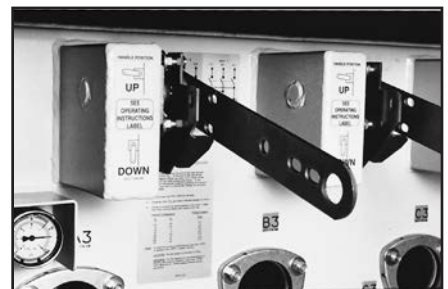
▲ Single phase interrupter operating handles.
