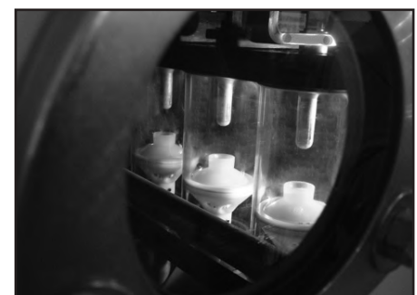
▲ Load break switch visible break.
