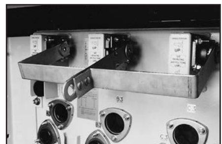
▲ Three phase interrupter operating handle.
