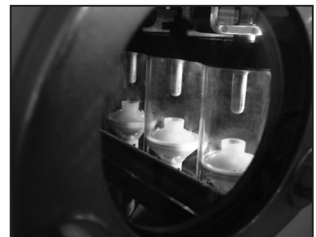
▲ Load break switch visible break.
