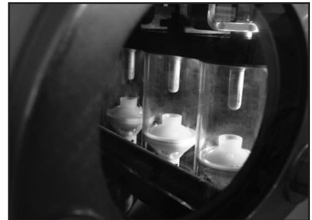
▲ Load break switch visible break.
