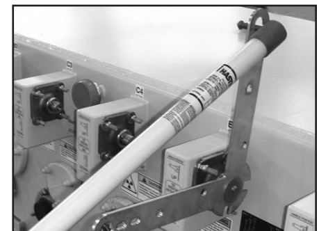
▲ Interrupter with dual operating handle.
