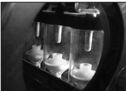
▲ Three phase visible position of contacts.
