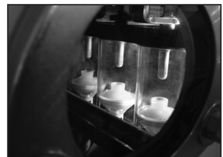
▲ Load break switch visible break.
