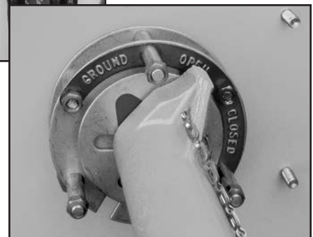
▲ Load break multi-position switch operator.
