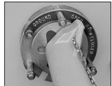
▲ Load break multi-position switch operator.
