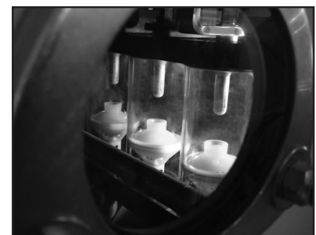
▲ Load break switch visible break.
