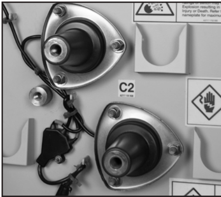
▲ 600A voltage sensing bushings
