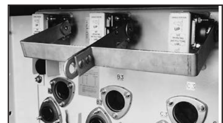
▲ Three phase interrupter operating handle.
