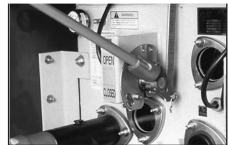
▲ Load break operating handle.
