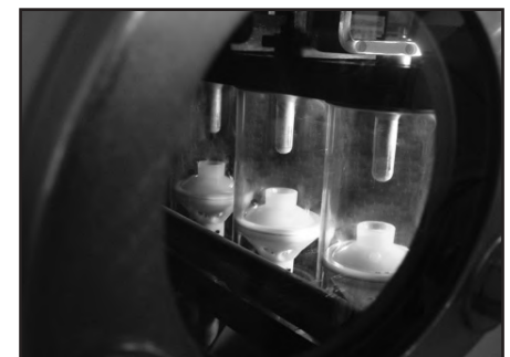
▲ Load break switch visible break.
