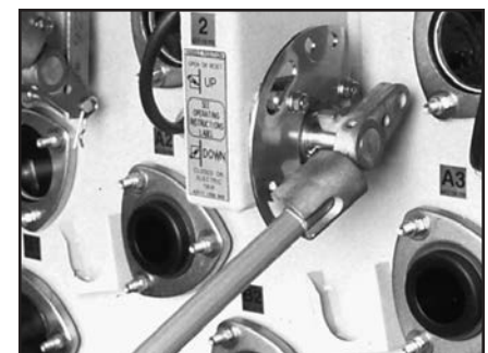
▲ Fault interrupter operating handle.
