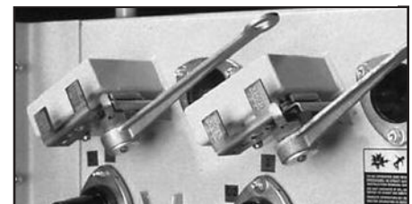
▲ Hookstick operable load break handle.
