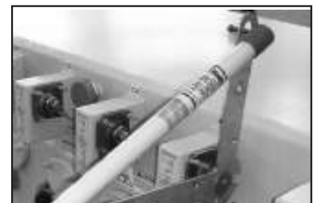
p Interrupter with dual operating handle.
