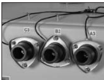
p 200A voltage sensing bushings
