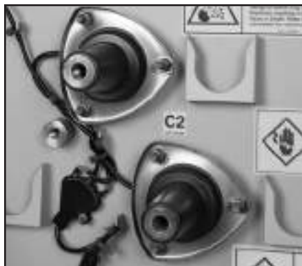
p 600A voltage sensing bushings
