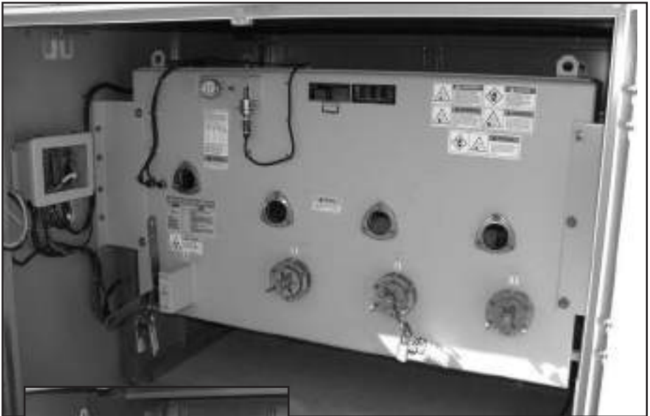
p Front and back view of a padmount PNI-43L with rotary style load break operator.
