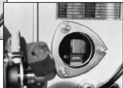
p Position indicators provide visible verification of contact position through viewing windows. u
