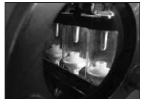
p Load break switch visible break.
