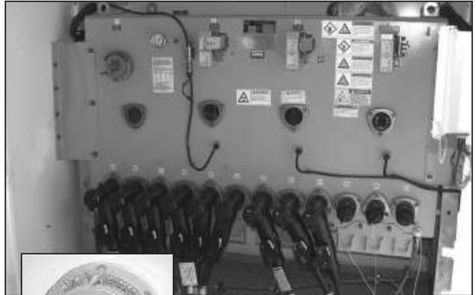
p Front access PNI with load break rotary operator and interrupter single operating handle.
