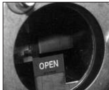
p Fault interrupter position indicator.
