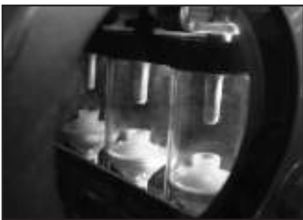
p Threephase visible position of contacts.
