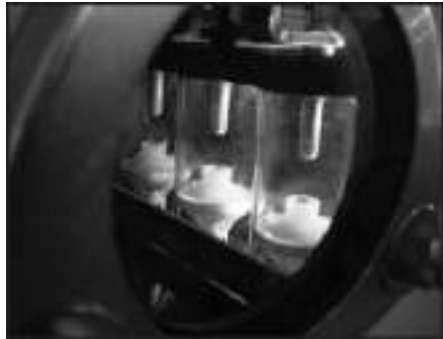
p Load break switch visible break.
