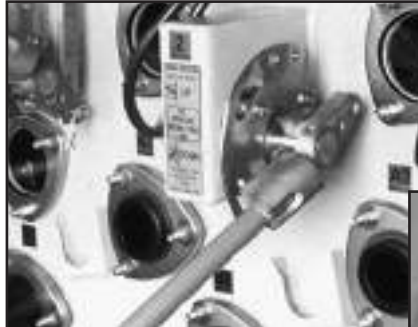
t Three phase interrupter operating handle for manual three phase operation and reset.
