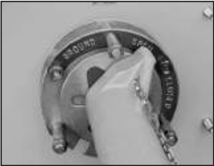
p Load break multi-position switch operator.
