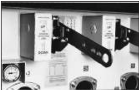
p Single phase interrupter operating handles.
