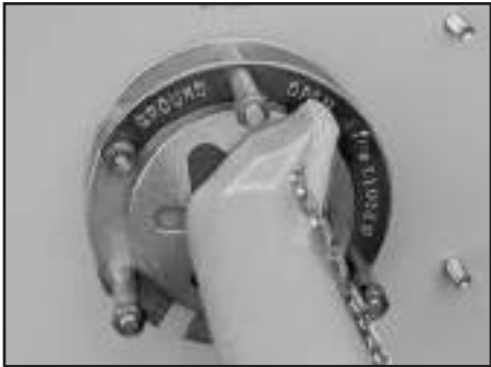
p Load break multi-position switch operator.
