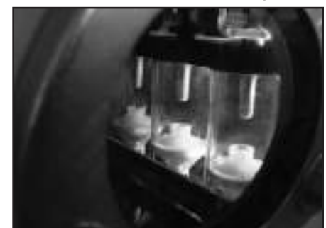
p Load break switch visible break.
