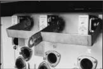
p Three phase interrupter operating handle.
