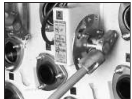
p Fault interrupter operating handle.
