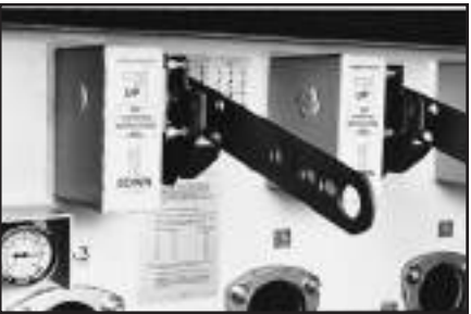
p Single phase interrupter operating handles.
