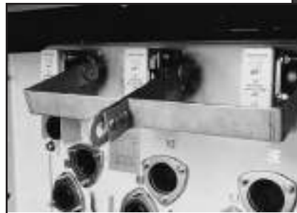
Position indicators (right) provide contact position indication through viewing windows.
