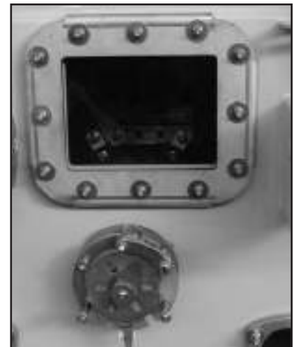
p Load break multi-position switch operator.
