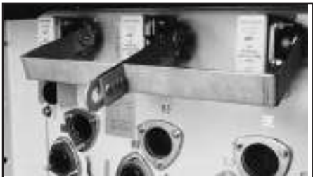
p Three phase interrupter operating handle.
