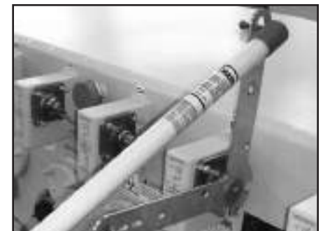
p Interrupter with dual operating handle.
