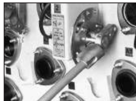
p Fault interrupter operating handle.
