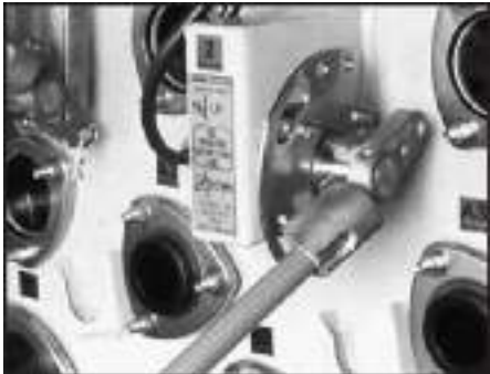
p Fault interrupter operating handle.
