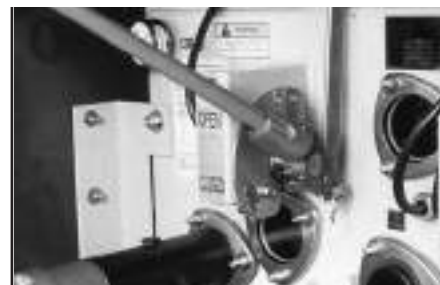
p Load break operating handle.
