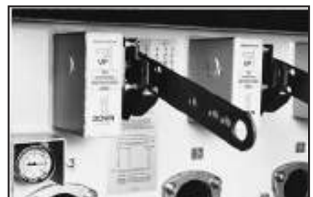
p Single phase interrupter operating handles.
