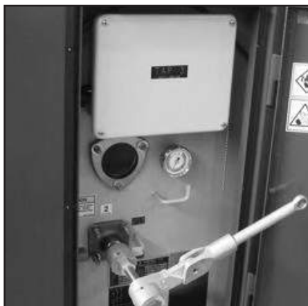
p All load break switch operators are located on the side of the switch.
