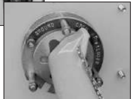
p Load break multi-position switch operator.
