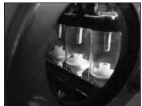
p Load break switch visible break.
